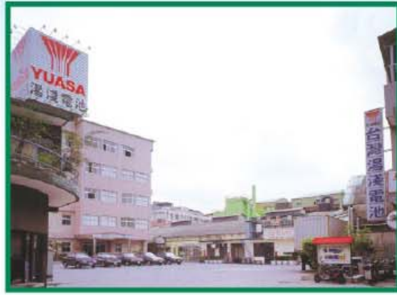
新莊廠 Hsin Chuang Plant
